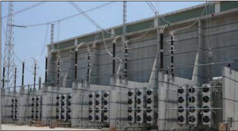
*Yidu HVDC Converter Transformers and Thyristor Building*
