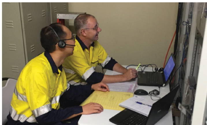
PSC team members Ken Choy (L) and Roger Ward at the Tennant Creek substation
